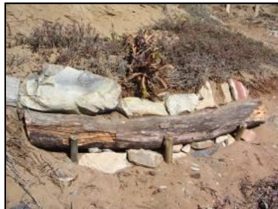
Damien at work repairing the soil erosion control measures.
