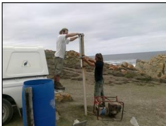
Roland and Damien re-erecting the old signage that had blown down.
