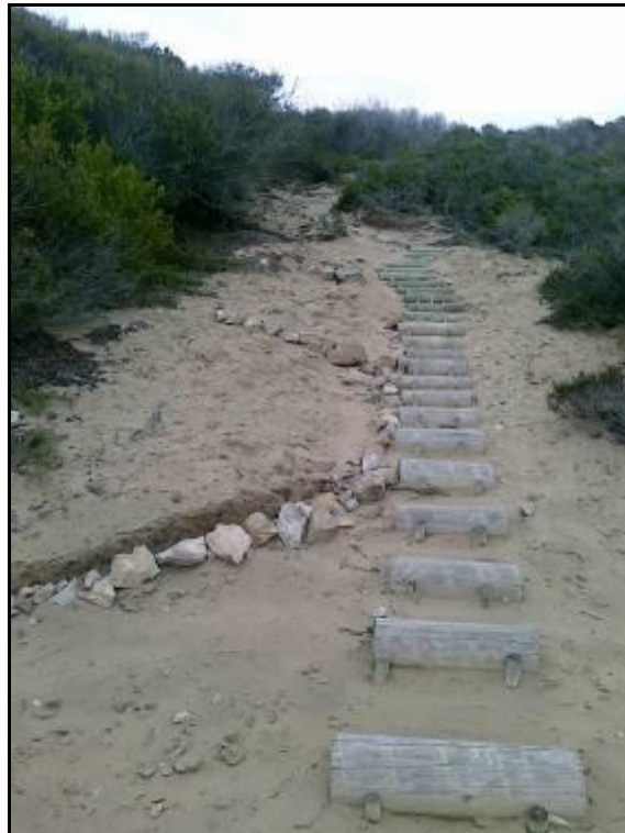
"Suicide Staircase", much easier to walk up after being repaired.
